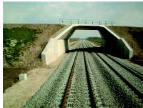
Figure 17: Construction element of nearly finished railway.
